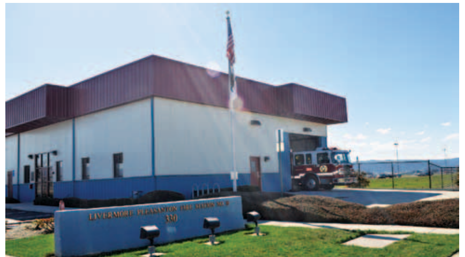
Fire Station 10 in Livermore is now reopened.
