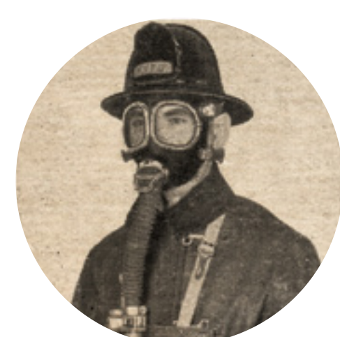
Outdated gas-mask canisters made way for more effective SCBA equipment thanks to efforts of local unions and CPF.
